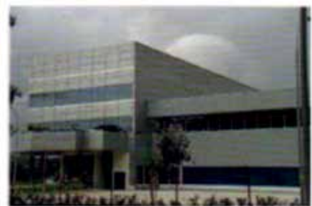
Caterpillar Building, Singapore
