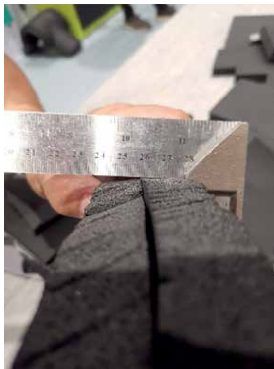
Improperly managed material can result in poor installation and inadequate insulation.
